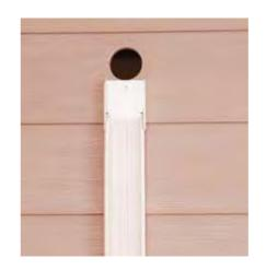
**Step 1**Fix the bottom parts of the fitting and the duct to the wall.
