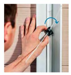
Place a cable tie in the SpinFix, insert and rotate the SpinFix onto the rail at the bottom of the SpeediDuct®.
