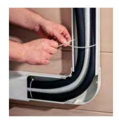
Lay the lineset, drain hose and controle cable inside the duct, strap the cable tie around them without damaging neither deforming them. Cut any excess of cable tie.
