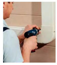
Install the fitting top (cover) for a rigid assembly using the included stainless steel screws.
