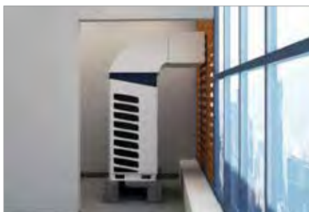
Installation du gainage.
